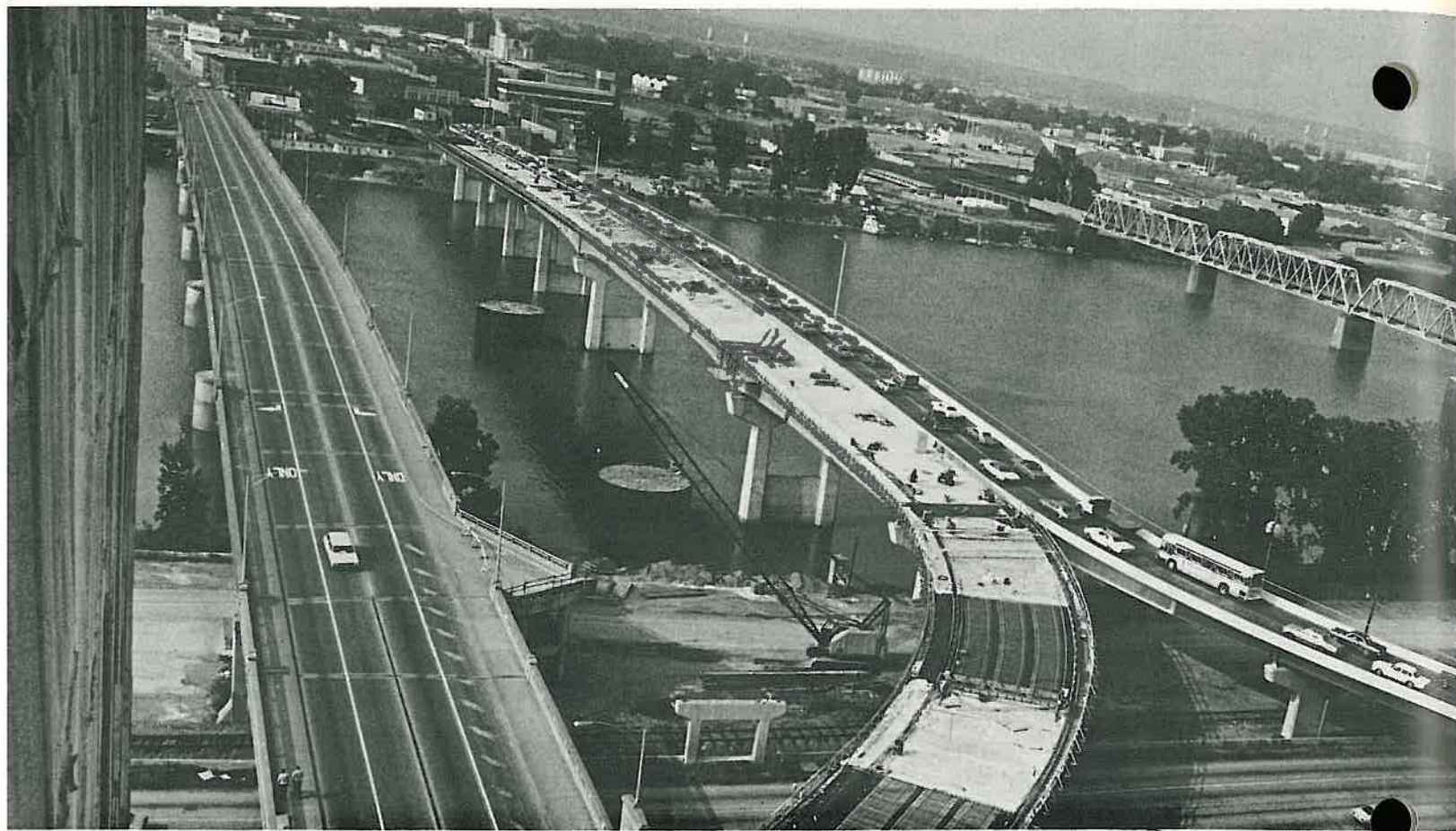
The old Main Street Bridge (left) and the new bridge, looking toward North Little Rock.
